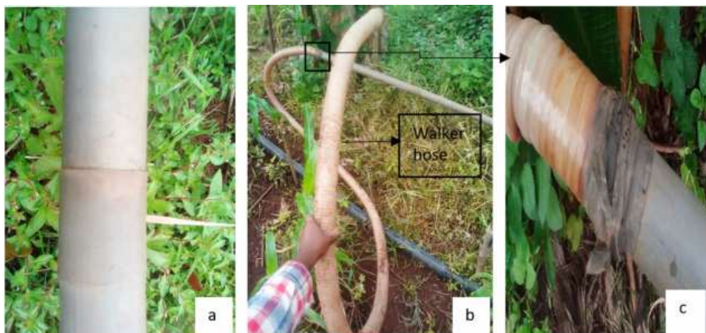
Fig. 4. System Components (a) Encased pipes (b) Walker hose connection (c) Rubber connection
