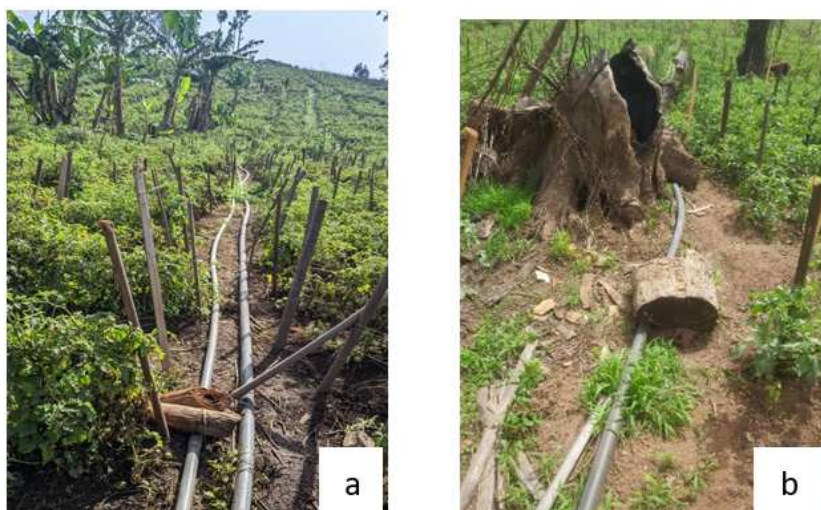
Fig. 5. Stabilizing the pipes (a) banana trunks (b) logs of wood
